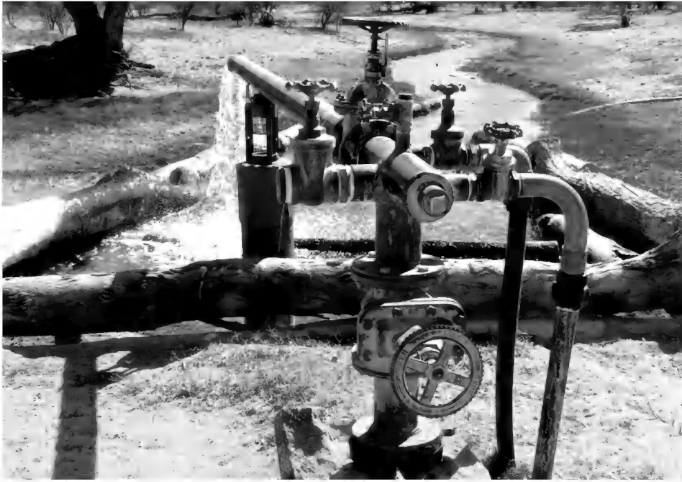
Figure 7. Open bore drains running from a controlled bore on a property near Julia Creek in Queensland (Source: GHD, 2019).
